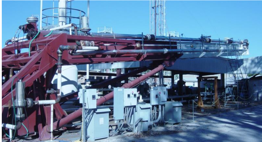
Figure 1: Photograph of the existing ACTF showing the base structure, mast and hydraulic cylinders
